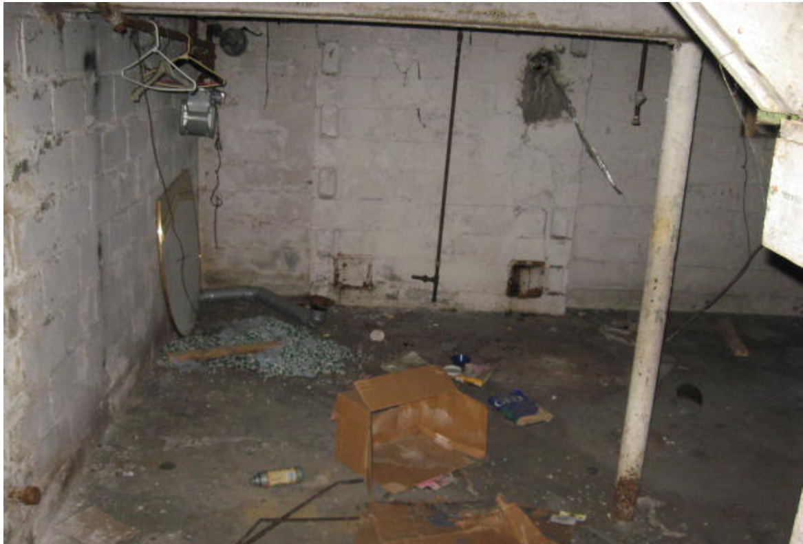
View of basement.
