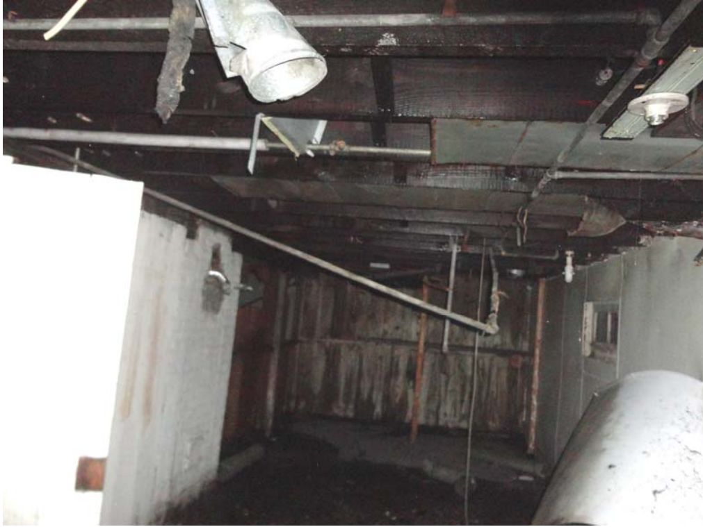
View of south basement.
