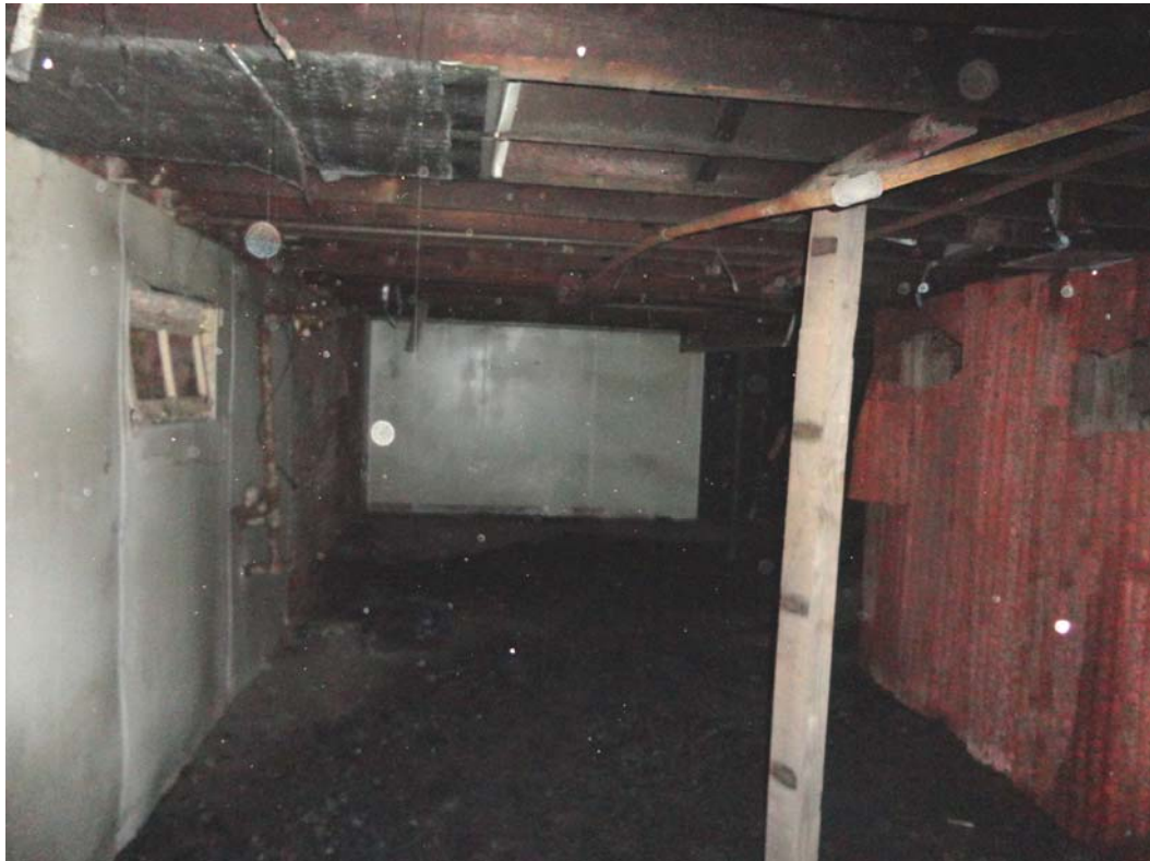
View of north basement.
