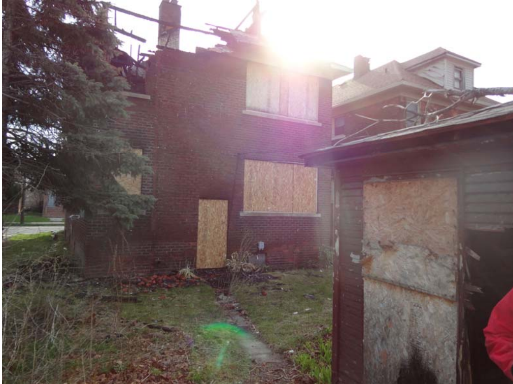
View of rear of the house from the alley.
