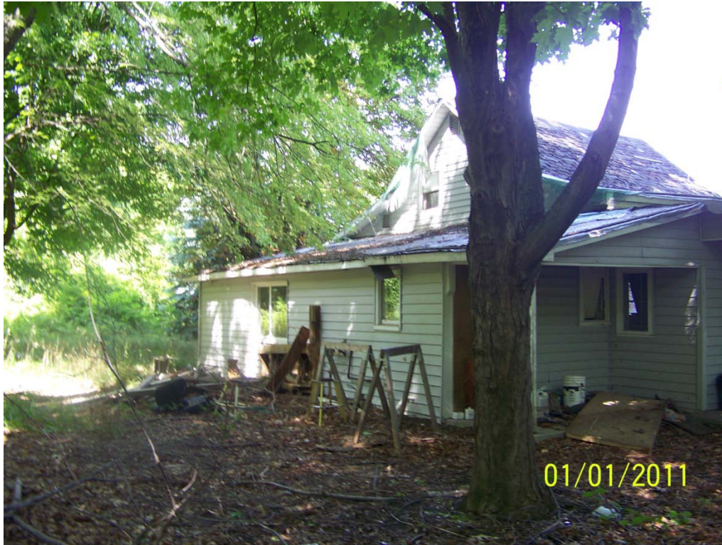
West side of home
