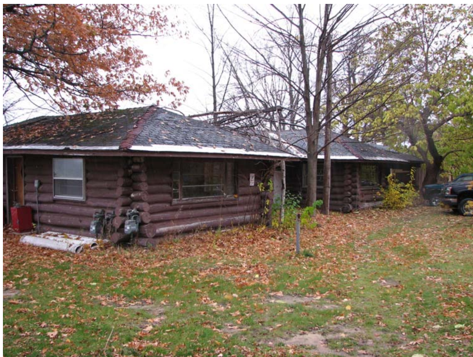
Residence viewed from the northwest with natural gas meters and pilings for a dock at the northwest corner
