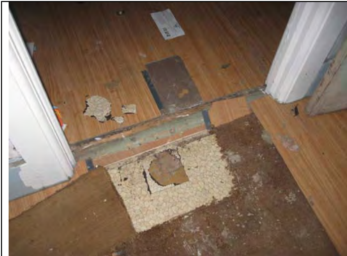
16. 1 st Floor Hall - linoleum (S-3 & S-4). The new snap-in surface flooring in the Foyer is not a SACM.
