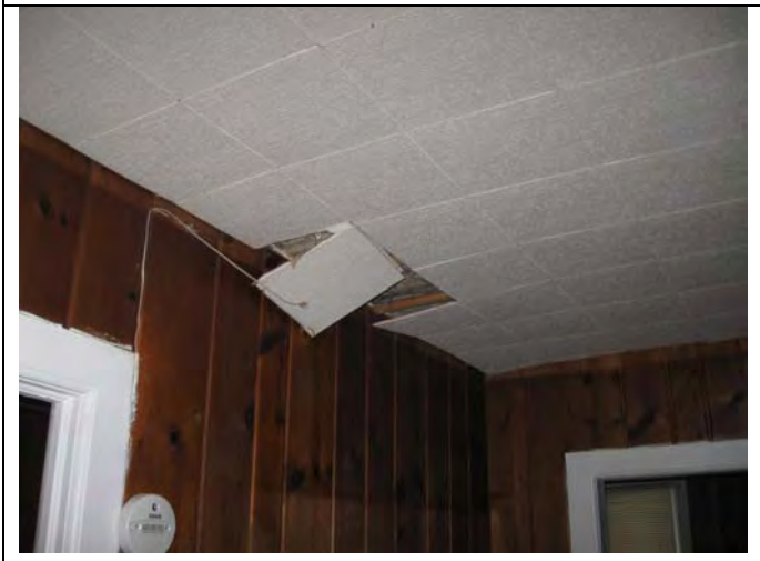
20. Dining Room - 12" x 12" ceiling tile (S-9) – nailed.
