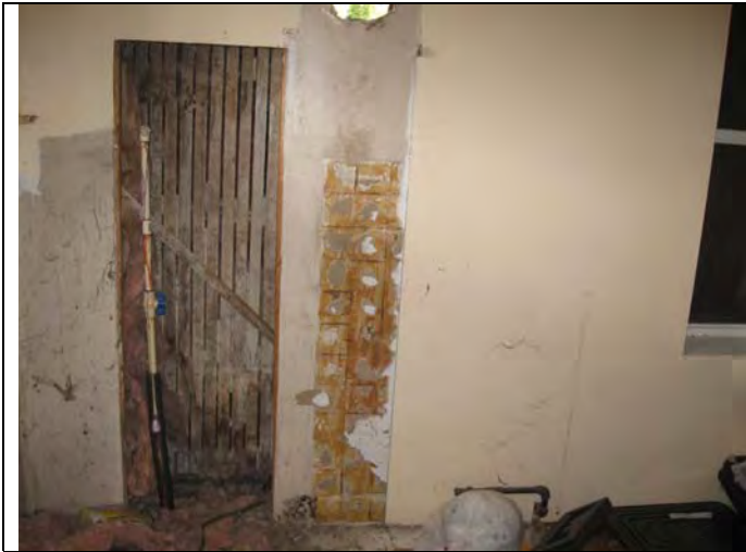
22. Kitchen – New drywall (S-11) was placed over the plaster.
