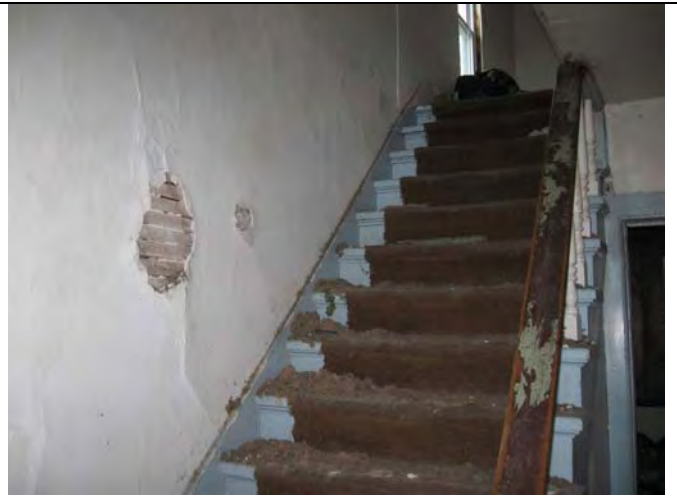
23. Plaster (S-12). Original finish on walls and ceilings.
