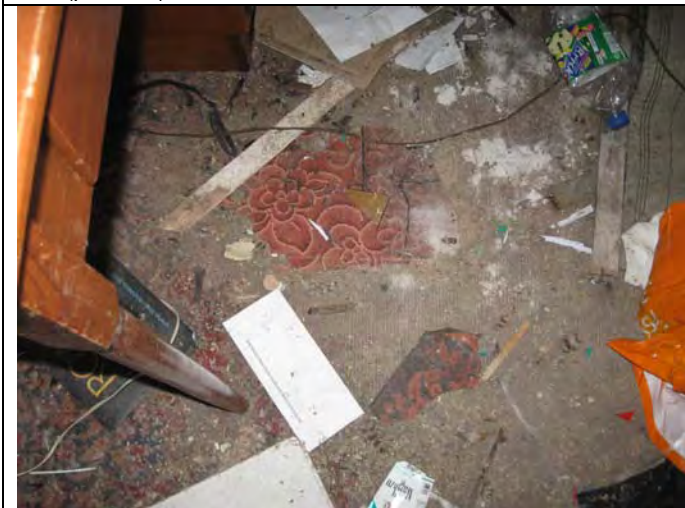
14. 2 nd Floor Landing - Linoleum (S-1)
