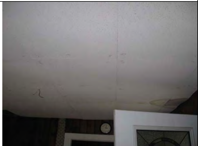
21. 1 st Floor Foyer – 2' x 2' ceiling tile (S-10) – new installation.
